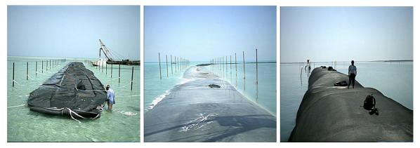
Figure 3-19 Example of Geotextile Breakwater Core Construction (Anwaj Is, Bahrain (Bergado, 2005))
